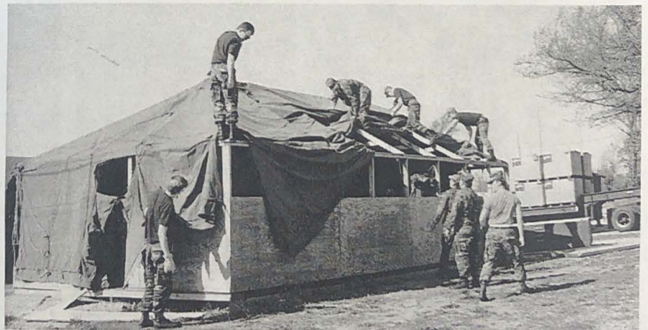
Civil Engineer crews prepare their "home for the night" by setting up this hard-back tent. (Photo by SSgt David C. Ellison)
